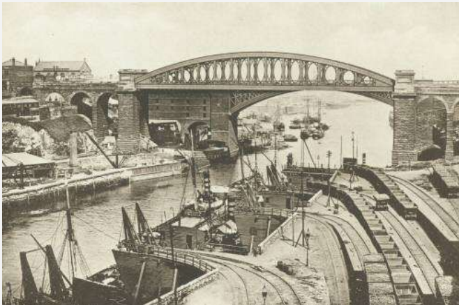
Fig : shipbuilding and industrial belts along the river bank.
